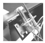
Again, being very careful, bring the copper conduit around from the thermocouple to the port on the back end of part 1 and connect it.
