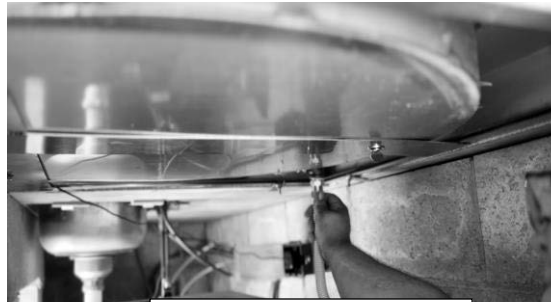
9- Tighten gas line to bottom of hearth
