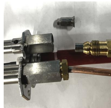
Figure 9.3 – Cleaning pilot orifice
