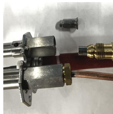
Figure 9.3 – Cleaning pilot orifice
