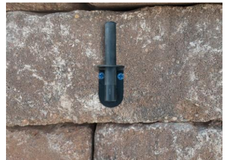
Figure 6.9 – Fasten down the bracket
