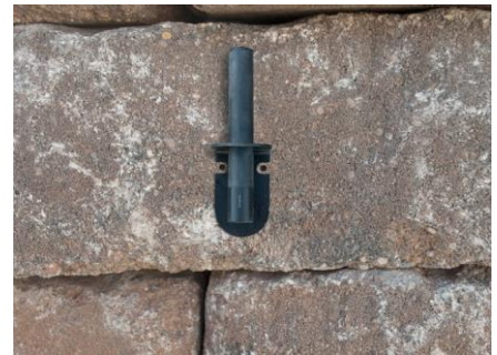
Figure 6.8 – Dry fit the bracket
