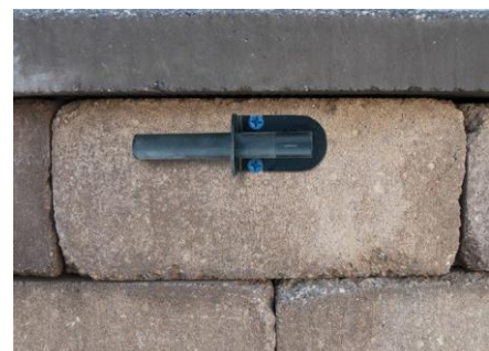
Figure 6.5 – Fasten down the bracket
