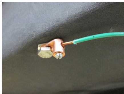
Bonding lug location for water only applications
