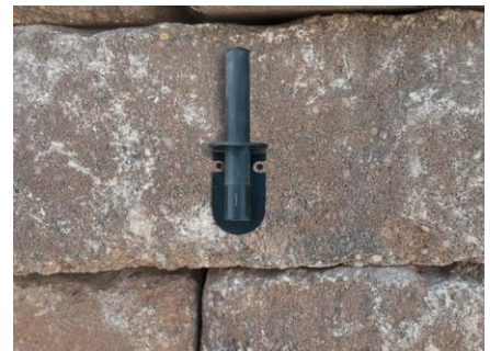
Figure 6.8 – Dry fit the bracket
