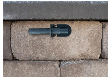
Figure 6.4 – Dry fit the bracket
