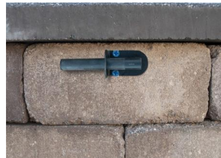
Figure 6.5 – Fasten down the bracket
