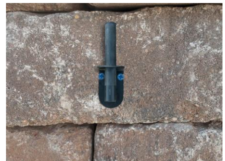
Figure 6.9 – Fasten down the bracket
