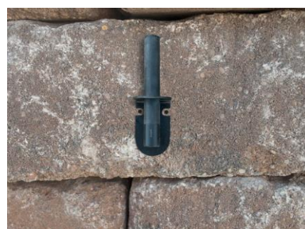
Figure 6.8 – Dry fit the bracket
