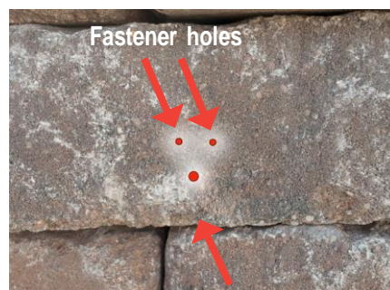
Figure 6.7 – Plot the hole locations
