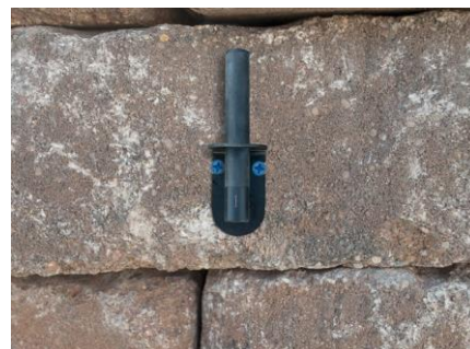
Figure 6.9 – Fasten down the bracket
