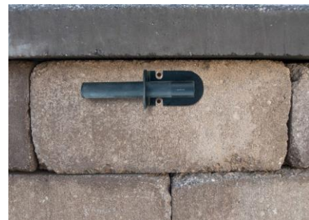
Figure 6.4 – Dry fit the bracket
